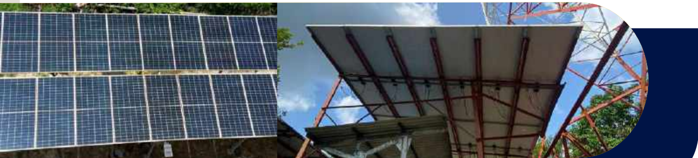
Telkomsel's BTS are equipped with solar panel.
